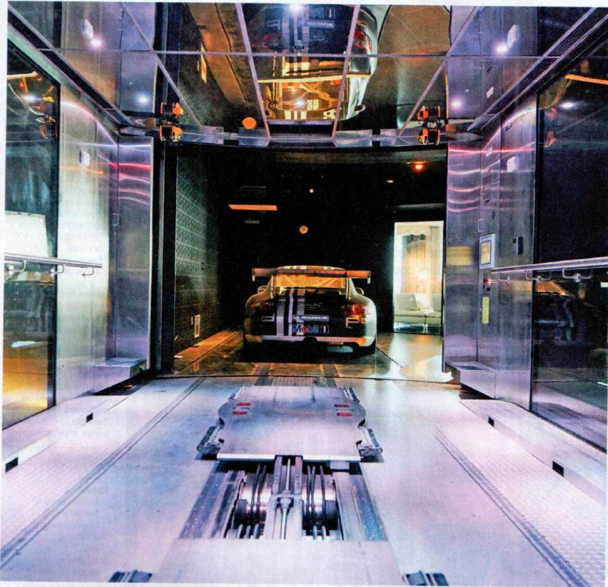
◀ Inside the elevator that whisks owners—and their cars—to apartments in the Porsche Design Tower in Sunny Isles Beach, Fla.
